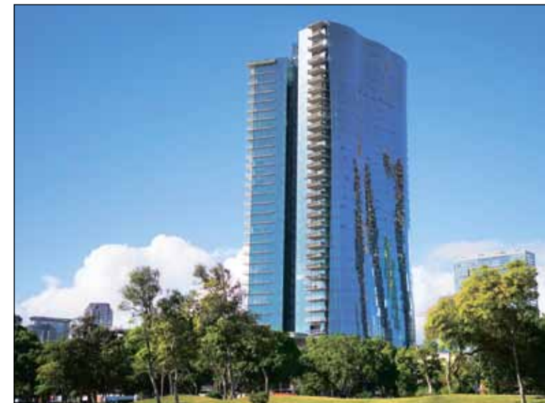
Waiea — with its sweeping, unparalleled glass facade and spacious view-oriented interiors, this 36-floor tower represents a level of architectural sophistication never before available in Hawaii.
